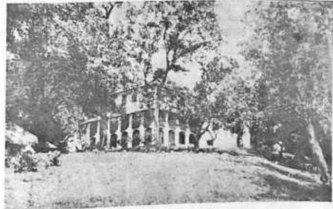
HERE WE BEGAN — THE THREE STORED BUILDING WHERE WE STARTED WORK
